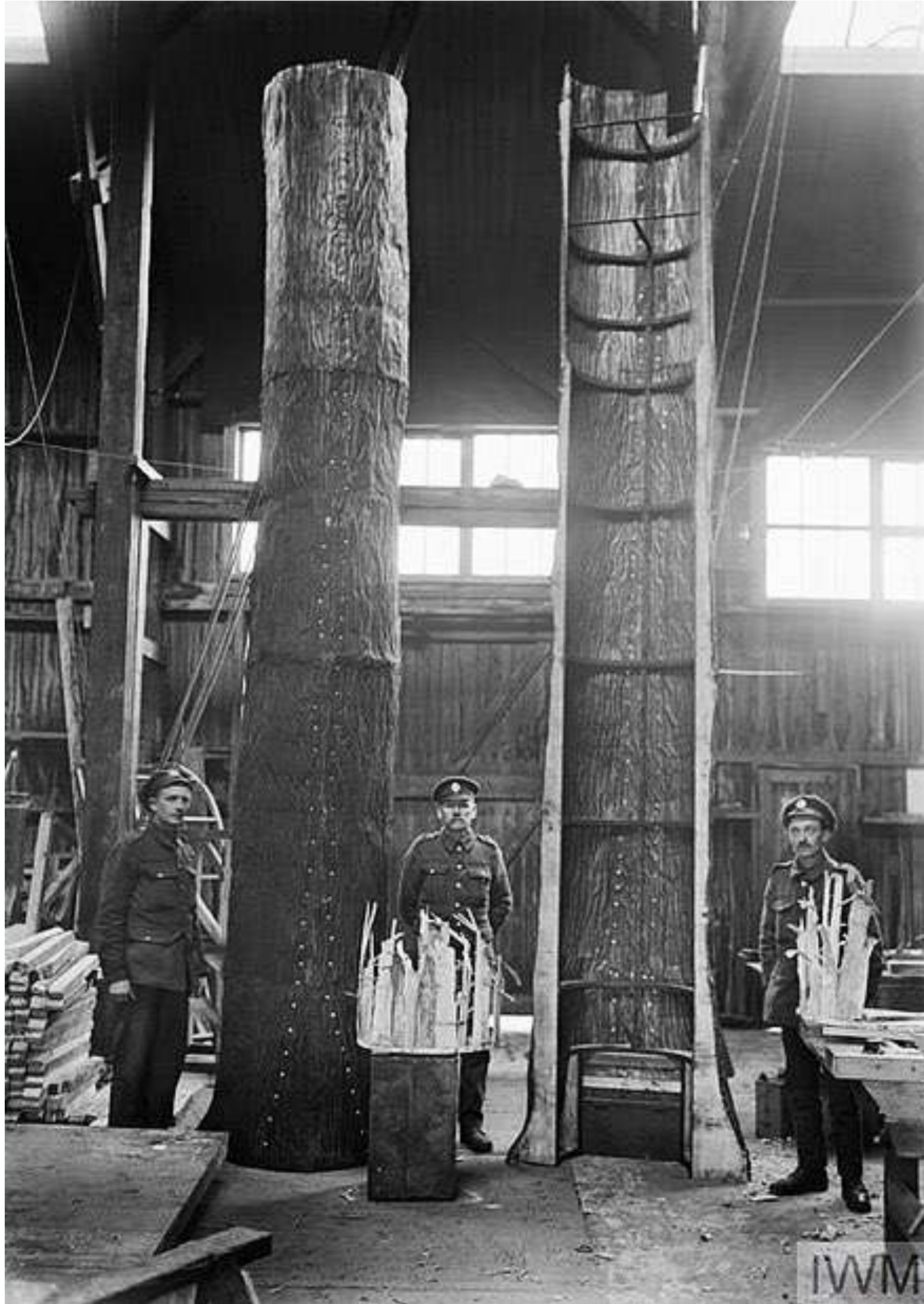
Production of a camouflage tree during WWI, France
